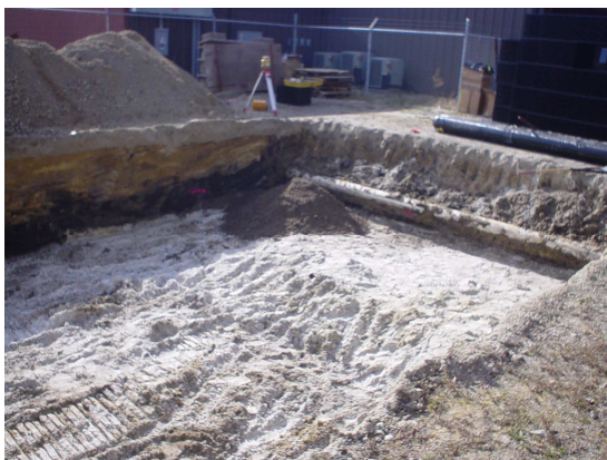
Site Prepared for Underground
